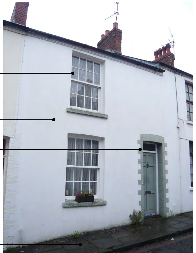
Two-storey terrace in a cottage style, late 19 th century.
