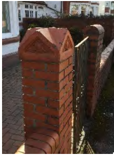
Brick pillars, decorative coping.
