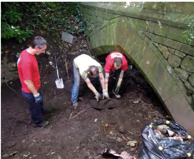
Prichard Bridge (2013) Restoration project.
