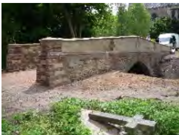
Prichard Bridge repair and refurbishment in 2012/13.
