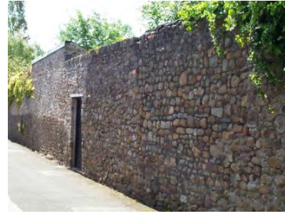
Historic rubble stone wall.
