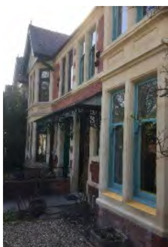
Cast iron and glass porches, Cardiff Road.
